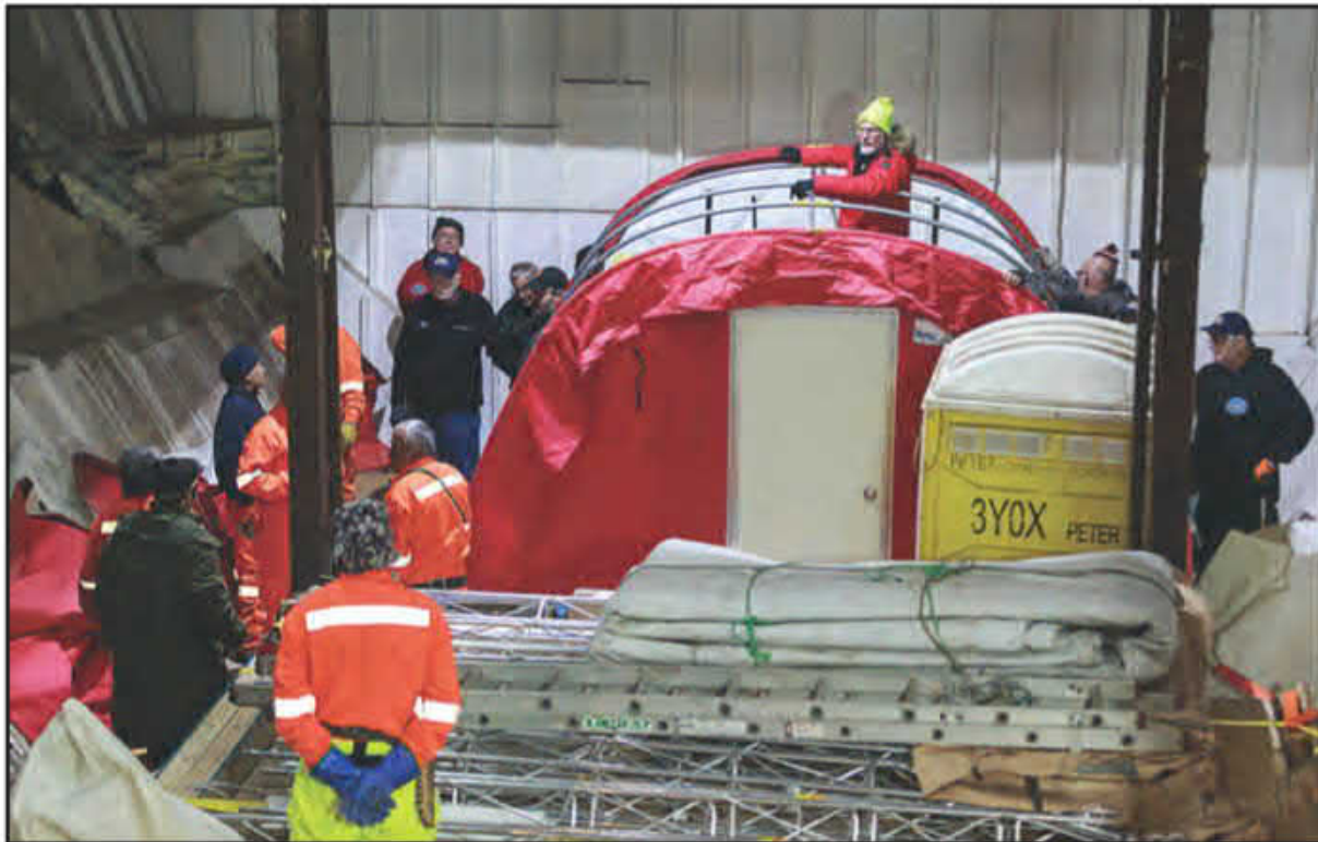
Shelter erection practice in ship's hold.
